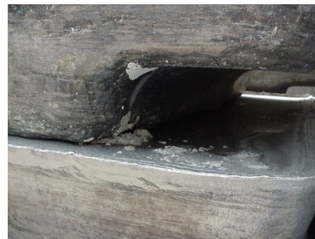
Figure 10: Release Agent Contamination
